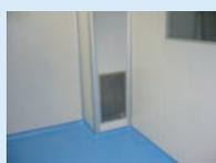
Stainless steel return grille with G4 filter included for integration at return air raisers (vertical or horizontal).
