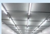
Tear drop lighting fixtures/luminaries, TL5 lamps, 58 W, for Laminar or Unidirectional airflow /weighting booths areas. Shape is specially designed to minimize disturbance to the airflow. IP20, CE mark.
